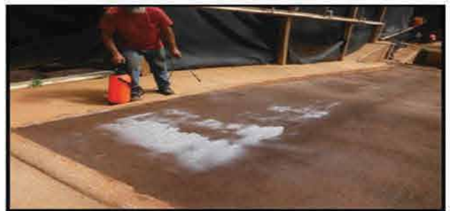
Mixture Sprayed at 1 gallon / 10 sf
